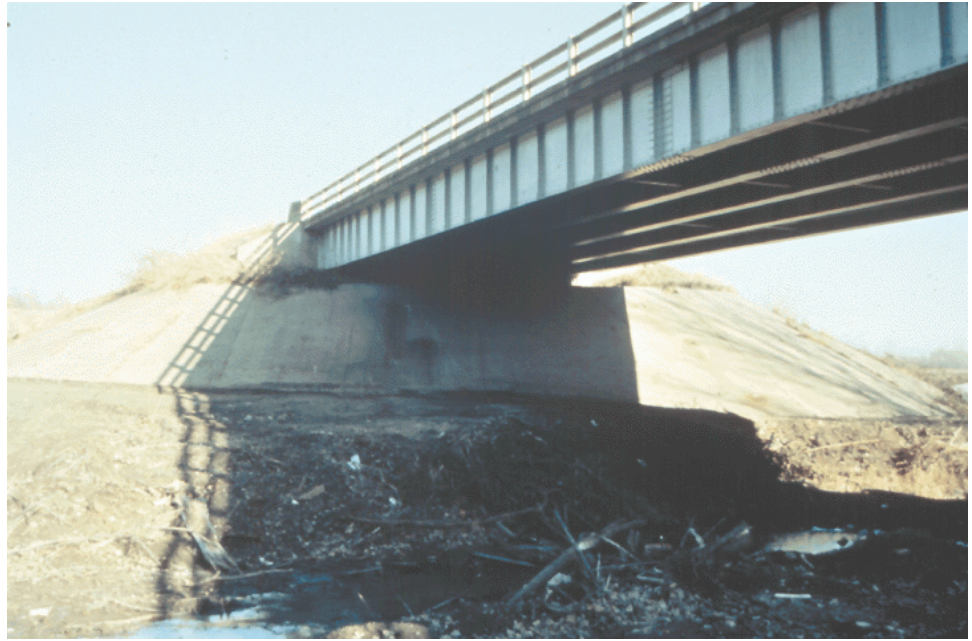
Figure 11.2.35 Approach Roadway Built in the Floodplain
