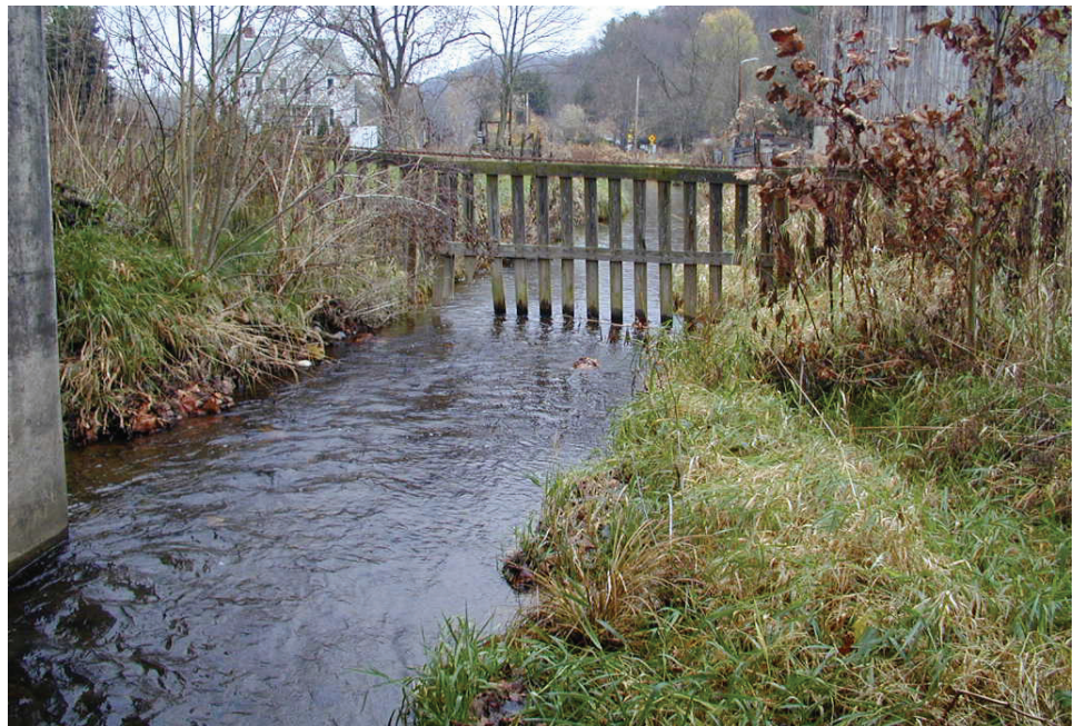
Figure 11.2.39 Fence in Stream at Bridge
