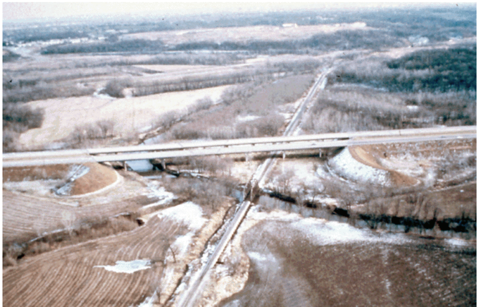
Figure 11.1.9 Guidebanks Constructed on Kikapoo Creek Near Peoria, Illinois
