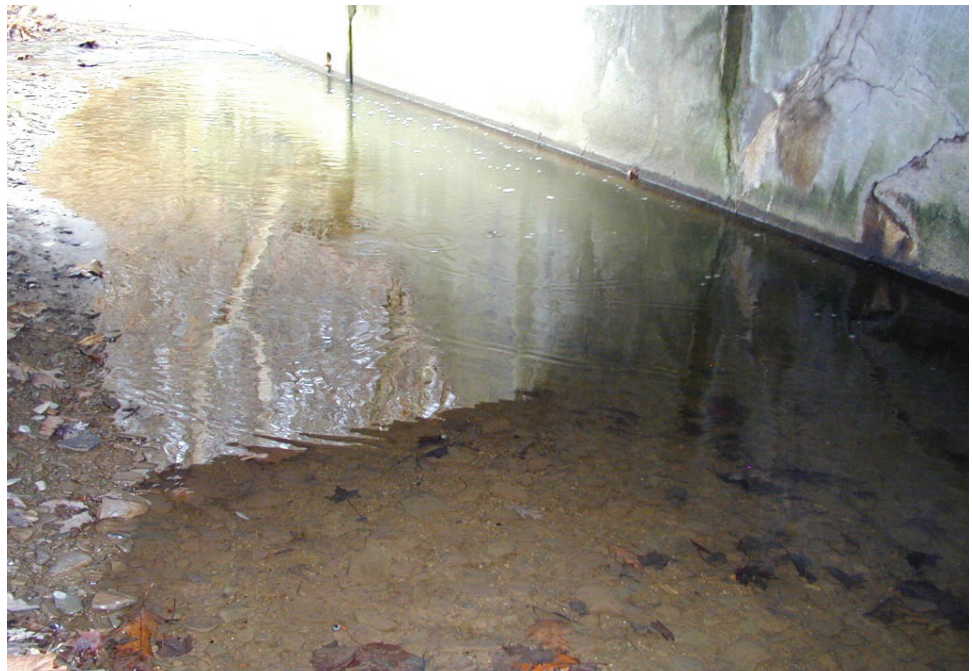
Figure 11.2.13 Local Scour at an Abutment
