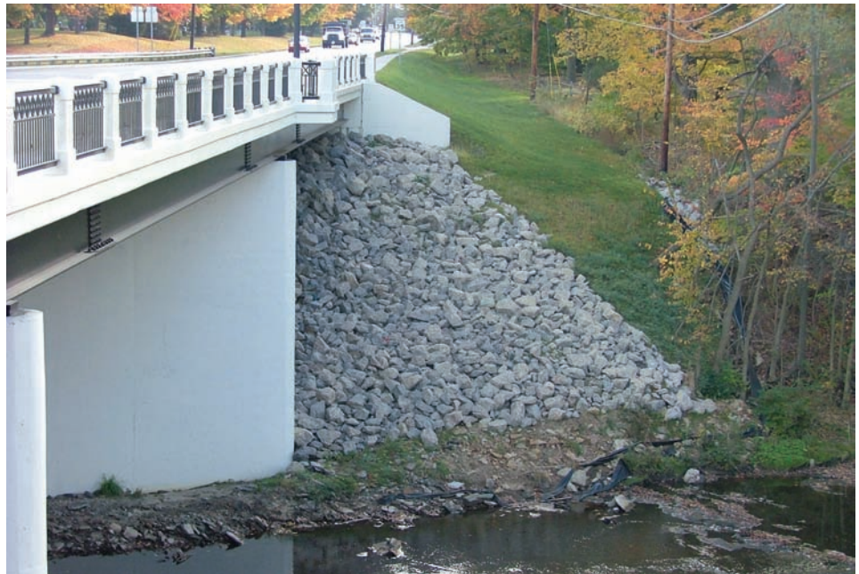
Figure 11.1.7 Crushed Stone Riprap
