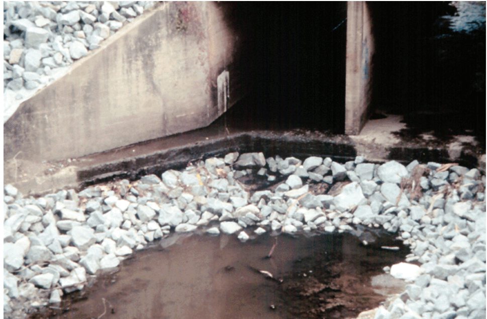
Figure 11.2.33 Failed Riprap
