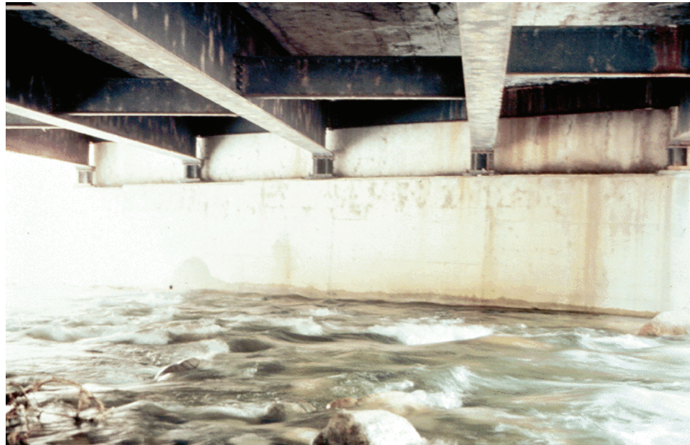
Figure 11.2.53 Accelerated Flow Due to Restricted Waterway
