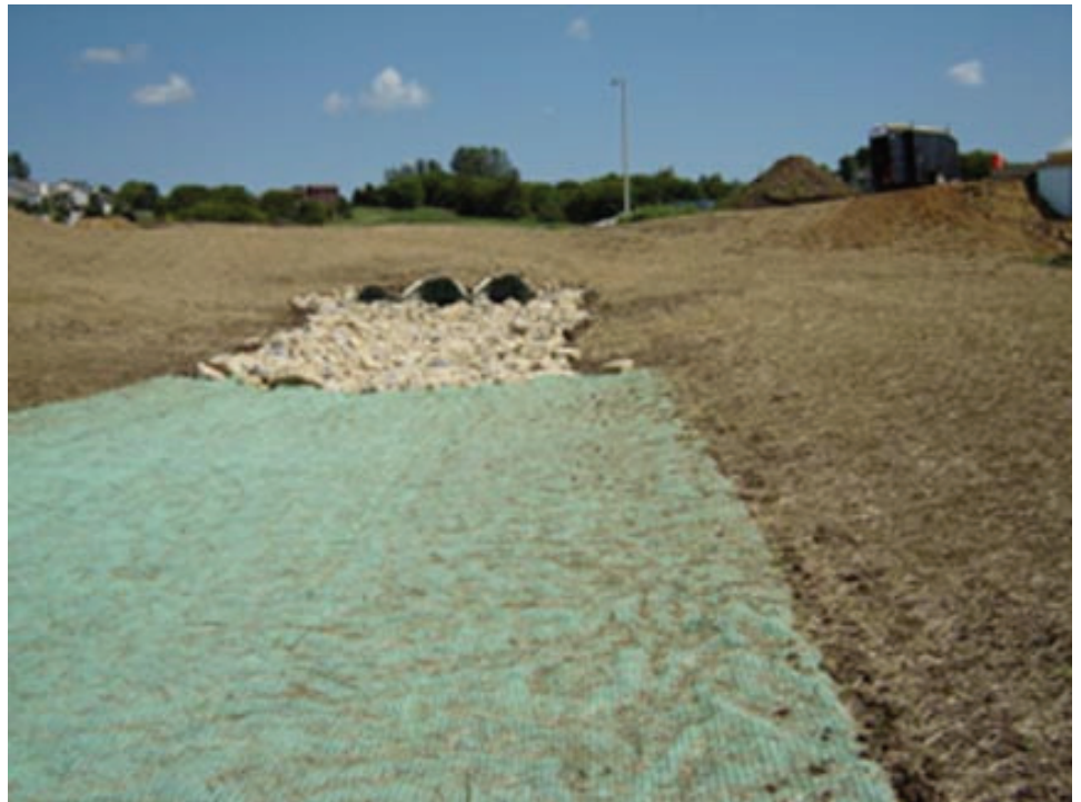
Figure 11.1.11 Wire Mesh and Grass Slope Stabilization
