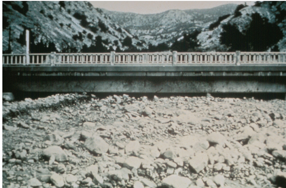
Figure 11.2.3 Streambed Aggradation
