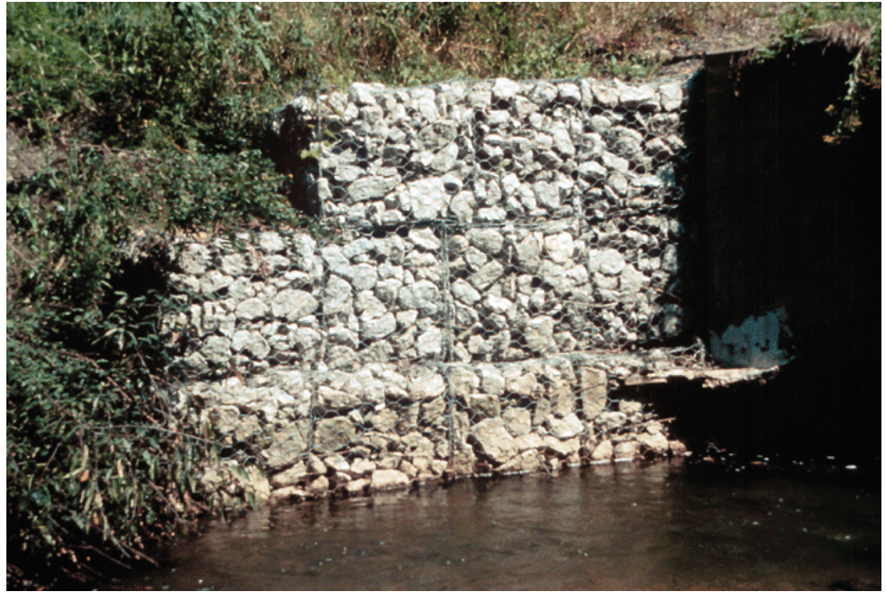
Figure 11.1.10 Gabion Basket Serving as Slope Protection
