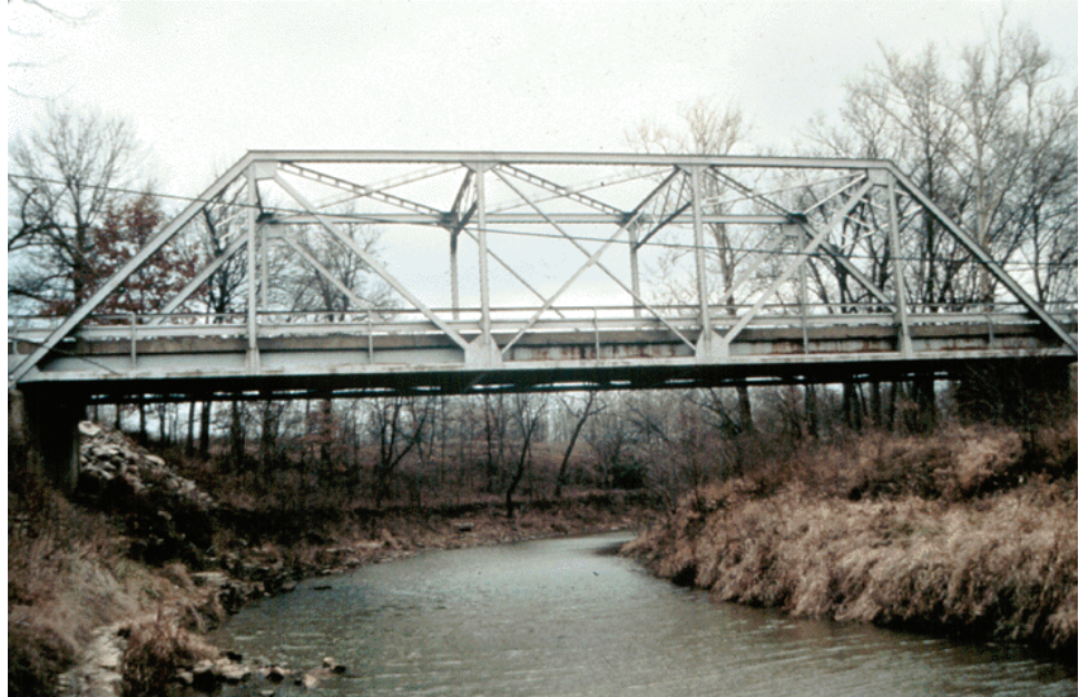
Figure 11.2.2 Streambed Degradation
