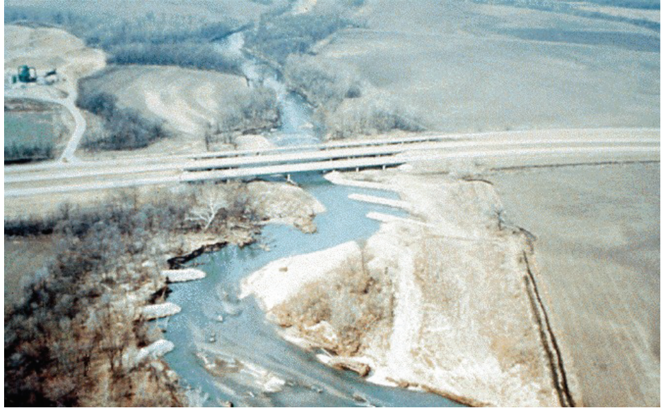
Figure 11.1.8 Spurs Constructed on Mackinaw River (Illinois Route 121)
