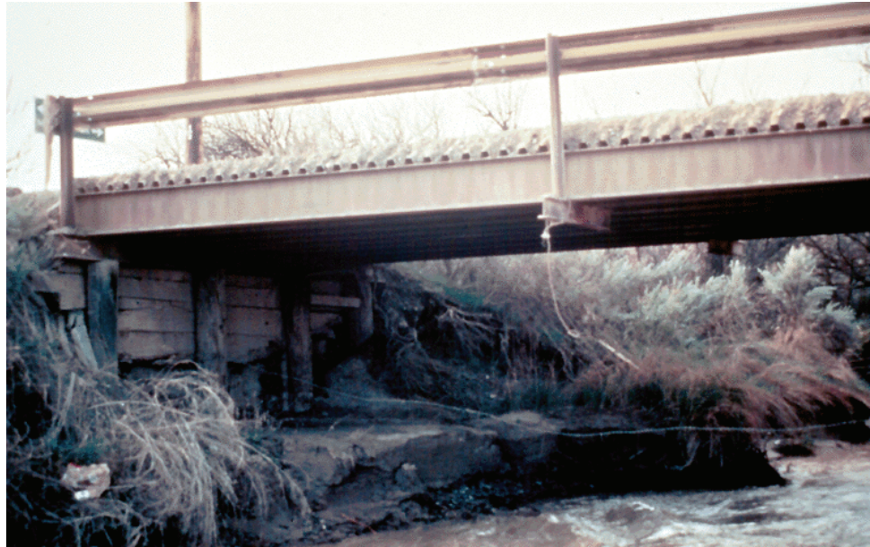
Figure 11.2.19 Channel Widening
