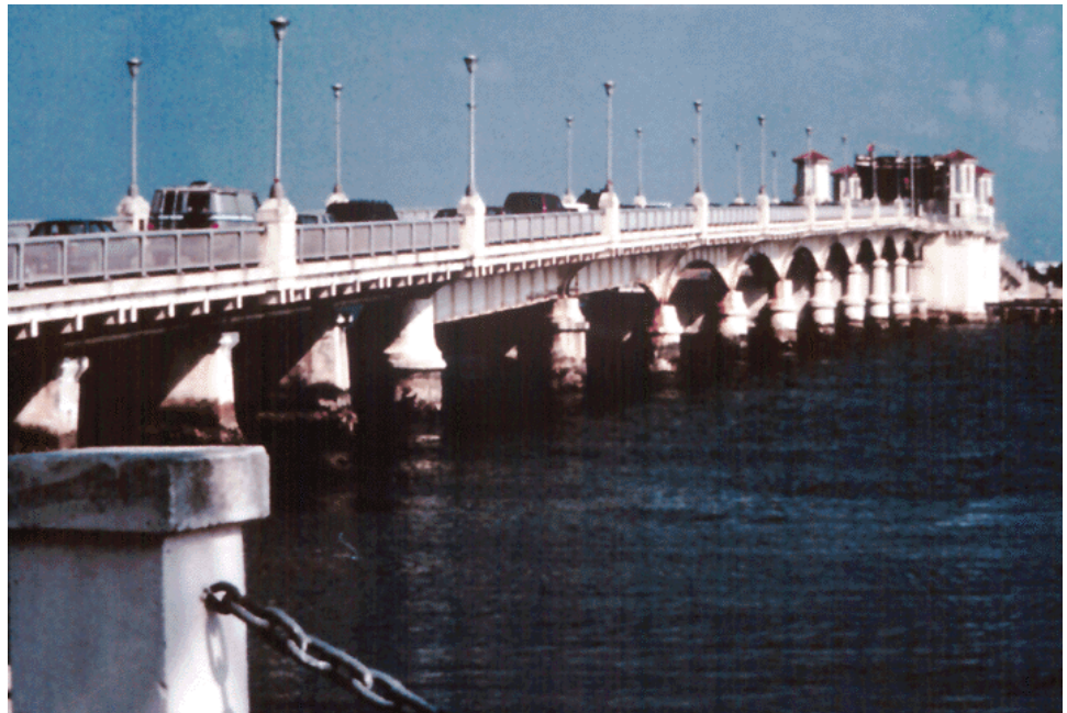
Figure 11.2.7 Large number of Piers Combine to Reduce the Hydraulic Opening
